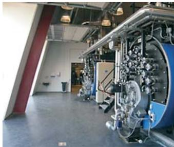
**The boiler plant** is a ble to supplement the solar heating with up to 5 kilowatt. The plant consists of two boilers that run on CO<sub>2</sub>-neutral biofuel. The plant has sufficient capacity to supply approximately 1,000 households with heating.
